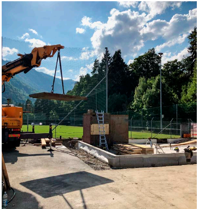
The measuring chamber was assembled using a heavy-duty crane. The image shows a steel element of the chamber ceiling being hoisted into place.
